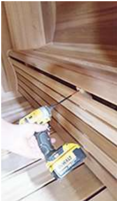
Screw the front enclosure and the bench seats together on the front tabs with 2 1/2" (64mm) screws.
