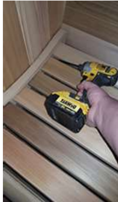
4 screws in each seat, 2 in front and 2 in the back. Screw between the seat boards to make the screws less visible.
